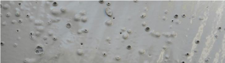
Blisters and or pinholes are most likely to be generated on hot, sunny days when the initial temperature of the substrate is relatively low, but increases rapidly due to heat generated from direct sunlight on the membrane.
