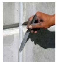
3. The final main feature of the backer rod is that is promotes an hour glass shape. This maximizes the bond area but keeps the depth of sealant consistent in the middle allowing for movement.
