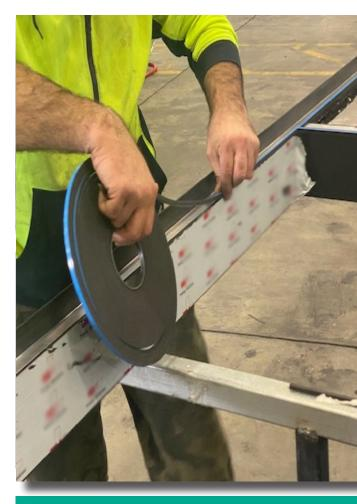
Designed to give a specific gap thickness for structural silicone in structural glazing systems.
