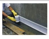
3. Overcoat VANDEX CONSTRUCTION JOINT TAPE with a second coat of VAN-DEX BB 75 E (minimum layer thickness is 2,0 mm) and smooth the surface with damp brush.
