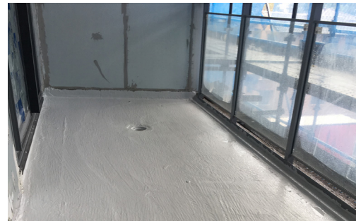
2. External Area - Tile and Screed
